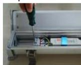
3. Connect the power cable to the right terminal through the cable gland
